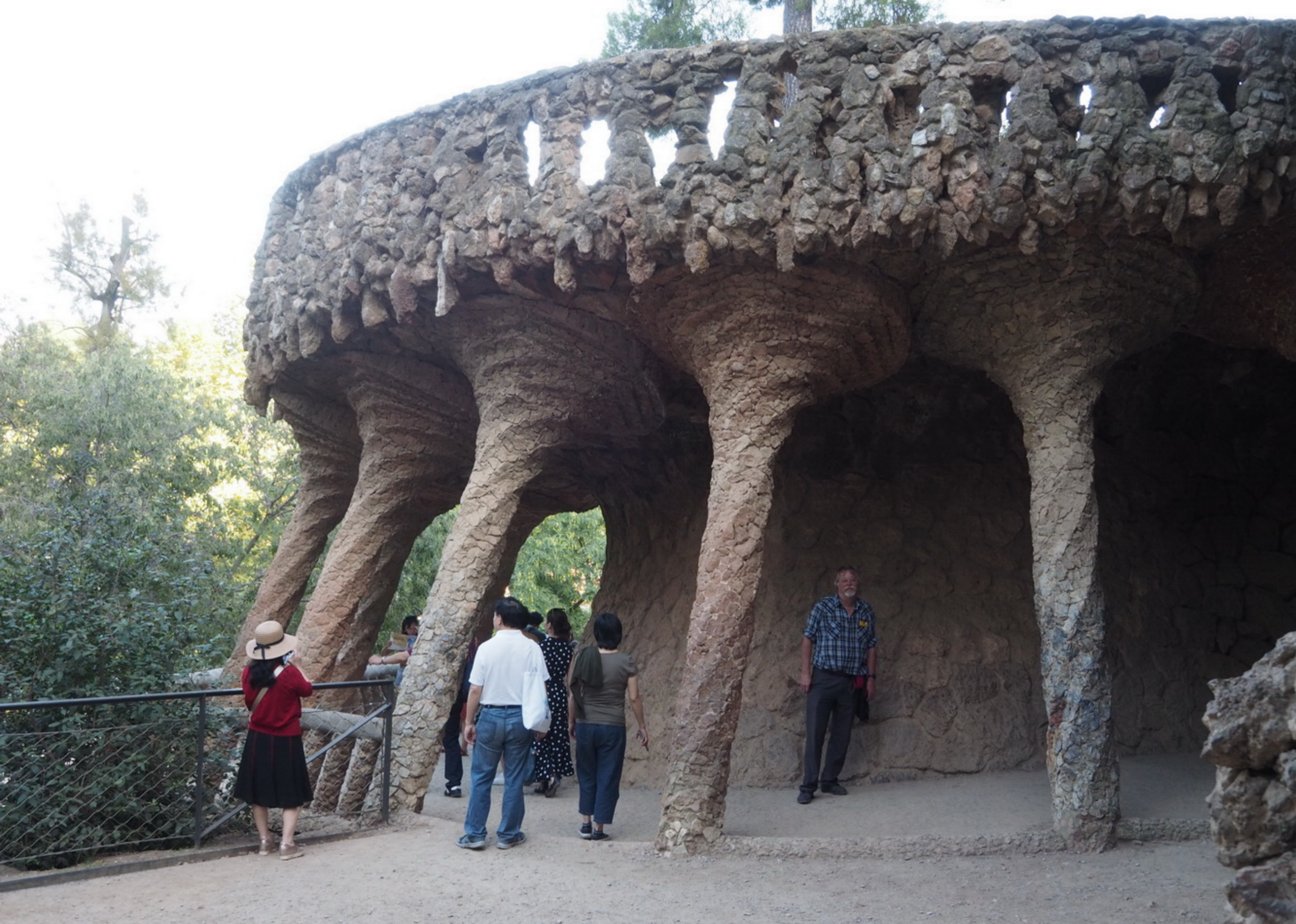
The "Pathway of Columns" supporting a viaduct.
